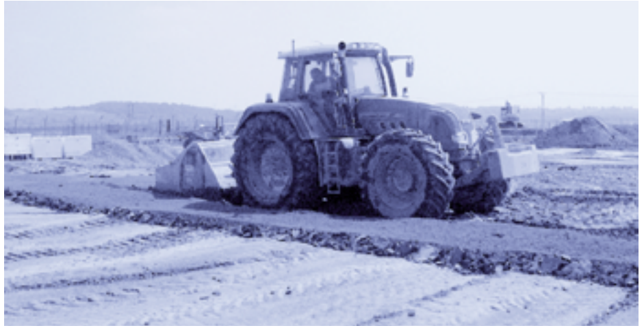
Incorporating PFA into the soil.
