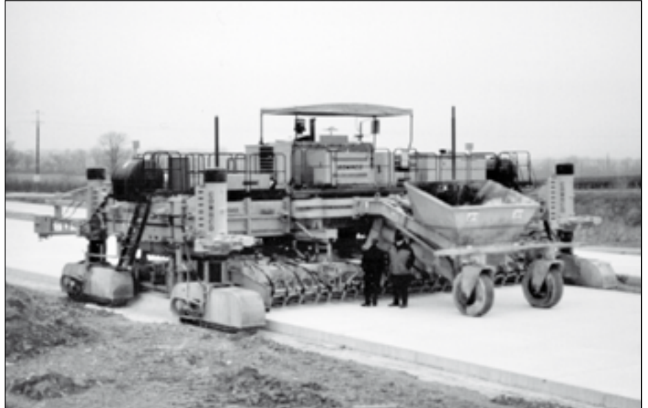
The Gomaco 4000 paving machine set at 10.75 m wide for this contract – stood down due to cold weather.
